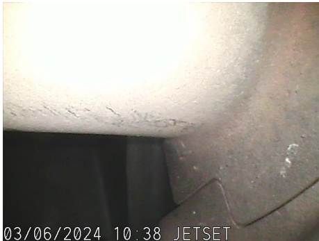
1 st Stage Low Turbine Blades
