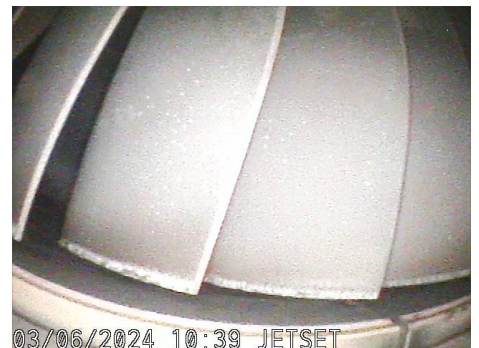
Aft Side of HT Blades
