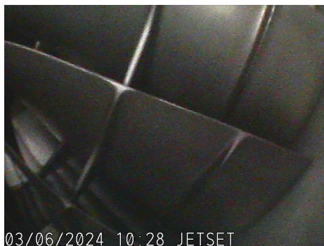
Low Compressor (Fan)
