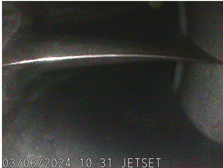
High Compressor (Impeller)
