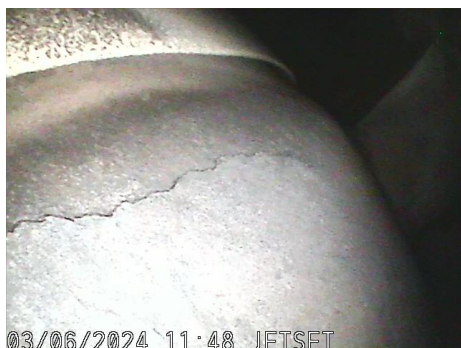
HT Vane Outer Wall Crack
